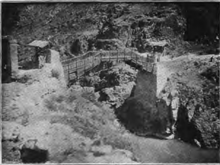
FIG. 5.—BRIDGE NEAR HSI-NING.
